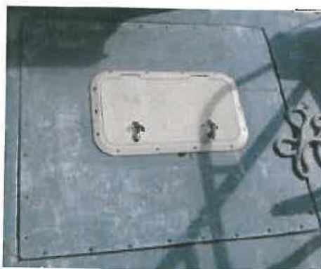
Lazarette deck plate, replaced as it had floated off after capsizing.
