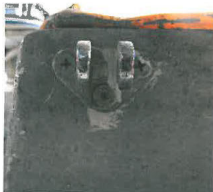
Coaming bracket installed.
