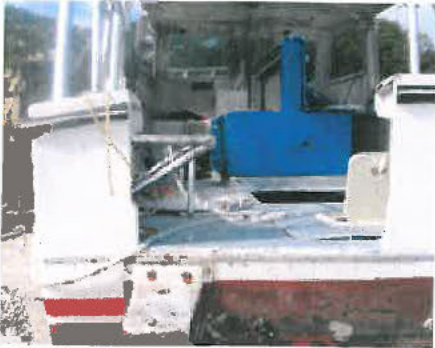
A section of the transom removed for divers' access to the swim platform
